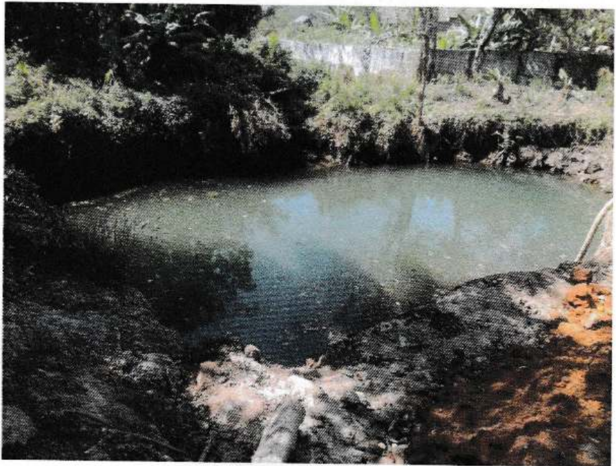
Annexure S-4: Rain Water harvesting pond
