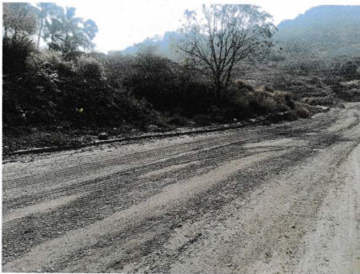
Plate G-15; Access road to the quarry.
