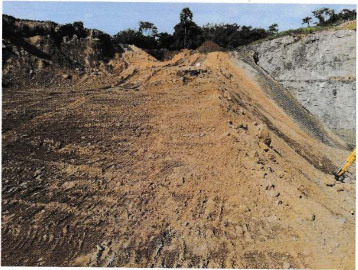
Plate G-16: Overburden is stacked
