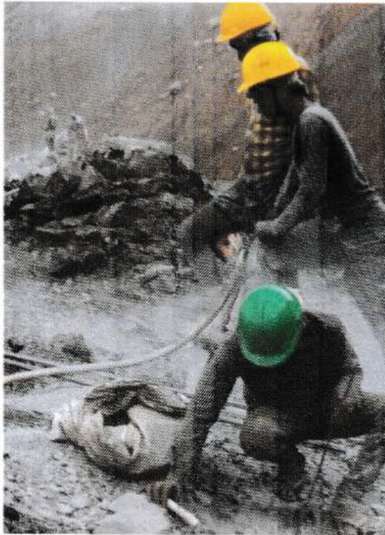
Plate G-22: workers with protective equipments
