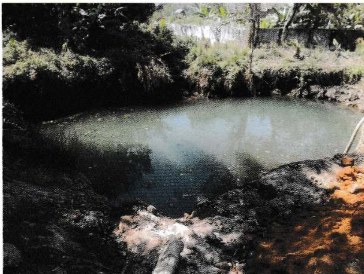
Annexure S-4: Rain Water harvesting pond
