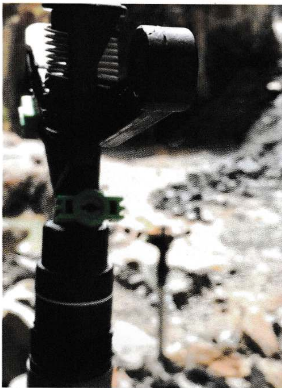
Plate G-5: Sprinklers
