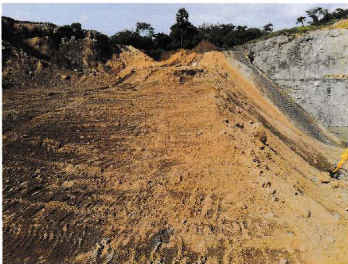
Plate G-16: Overburden is stacked
