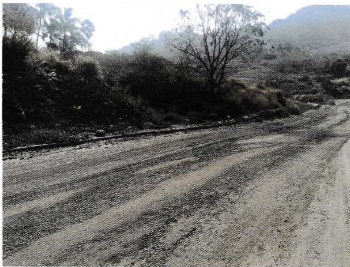
Plate G-15; Access road to the quarry.
