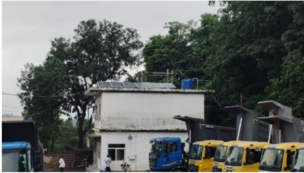
Fig 5: Photograph showing solar panel installation
